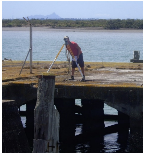
Leveling for tidal observations Limestone Island wharf – Portland channel Whangarei
